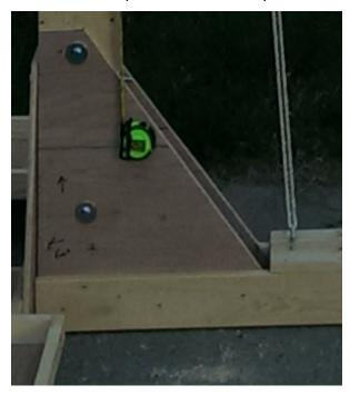
Drill 4 holes at the corners of the tape measure, and secure it in place with zip ties.
