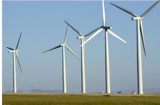
Fig. 3 Horizontal-axis turbines
