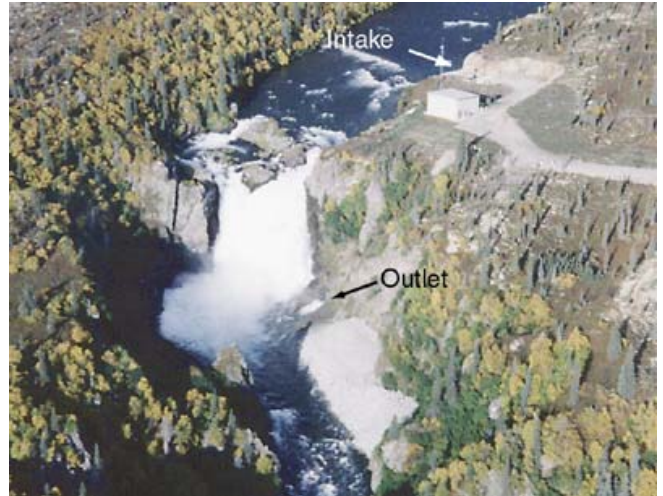
A diversion facility at Idaho Falls.
